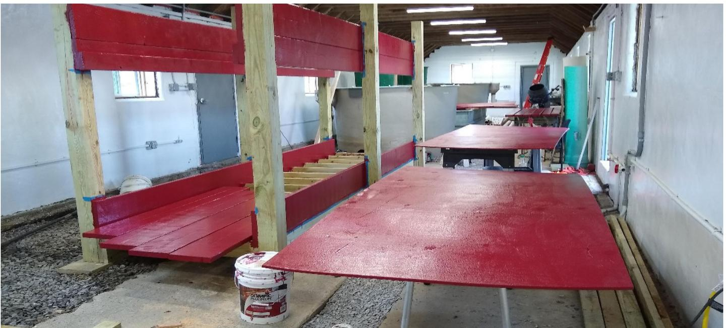
*Progress on one of the two deep-water aquaculture growing beds. Behind the two growing beds are the tanks; not seen are the sediment filters, biofilters, and oxidation tank. In the front bottom of the picture is the platform for the vertical growing system.*
